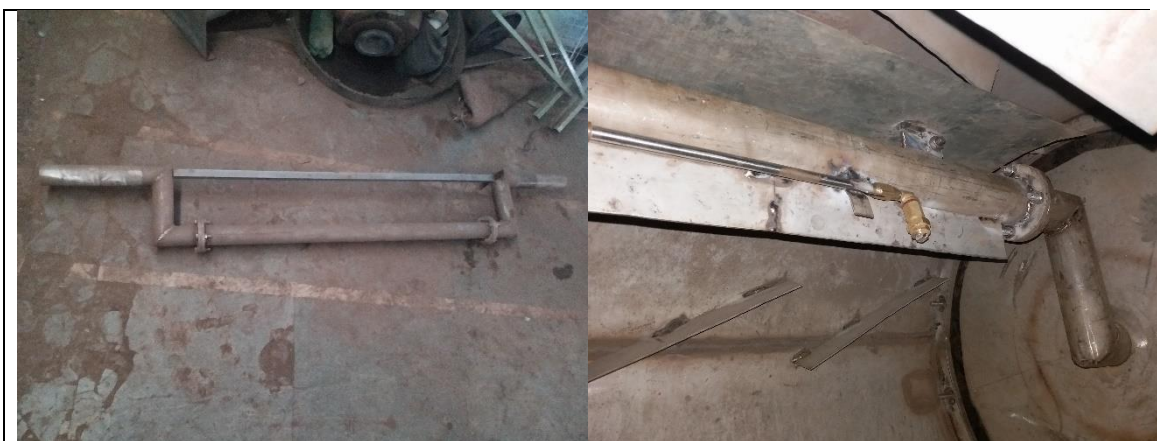
Plate 3.7 Fitting of centre shaft assembly of the drum
