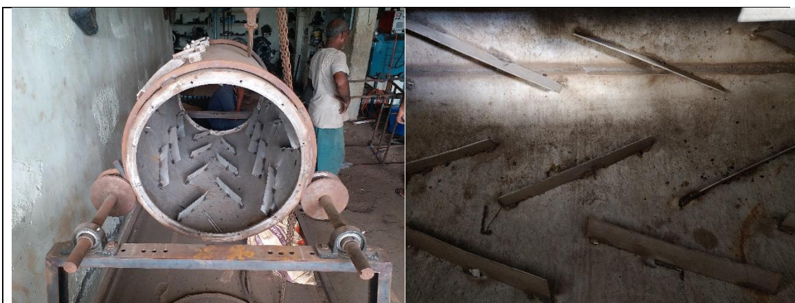
Plate 3.6 Fitting of flights inside the drum
